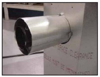
**Figure 9.10** Attach the first vent section (it will snap into place). Slide the insulation gasket onto the vent section, up against the appliance and over the tabs.
